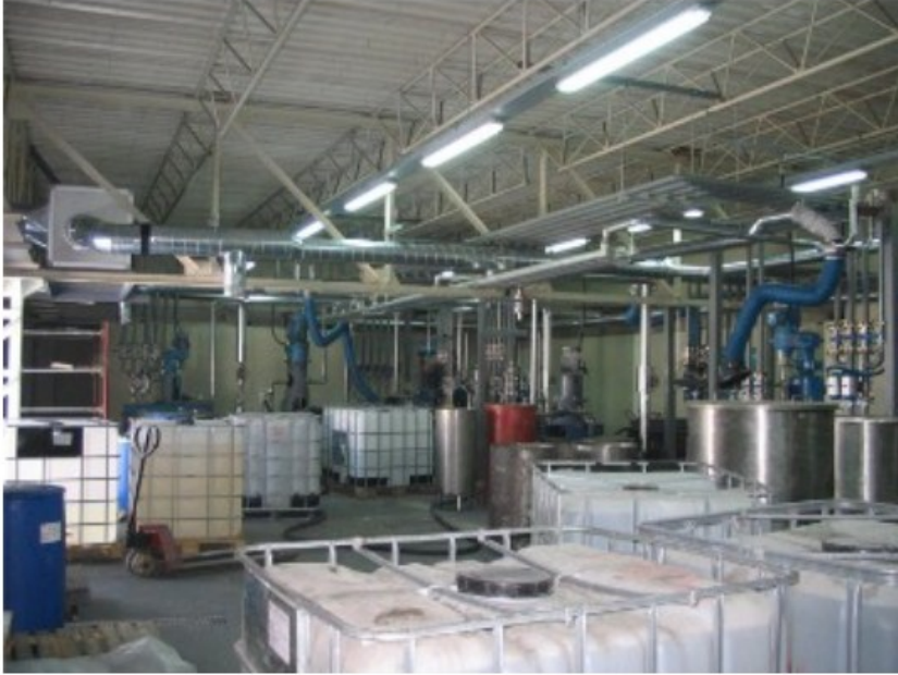
CHT TEKSTİL KİMYA SAN. TİC. A.Ş. Miscellaneous gas elimination systems
