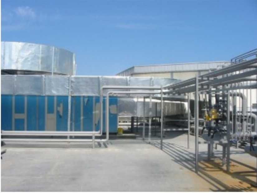
Kale Shopping Center Heat insulation application
