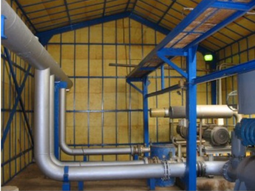
Akkim Kimya San. A.Ş. Yalova Plant Blower sound insulation application
